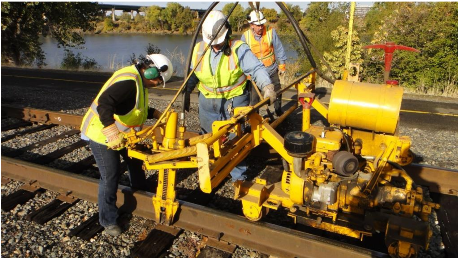
Pam and Heather use the hydraulic spike-puller to pull spikes on the ties being removed
