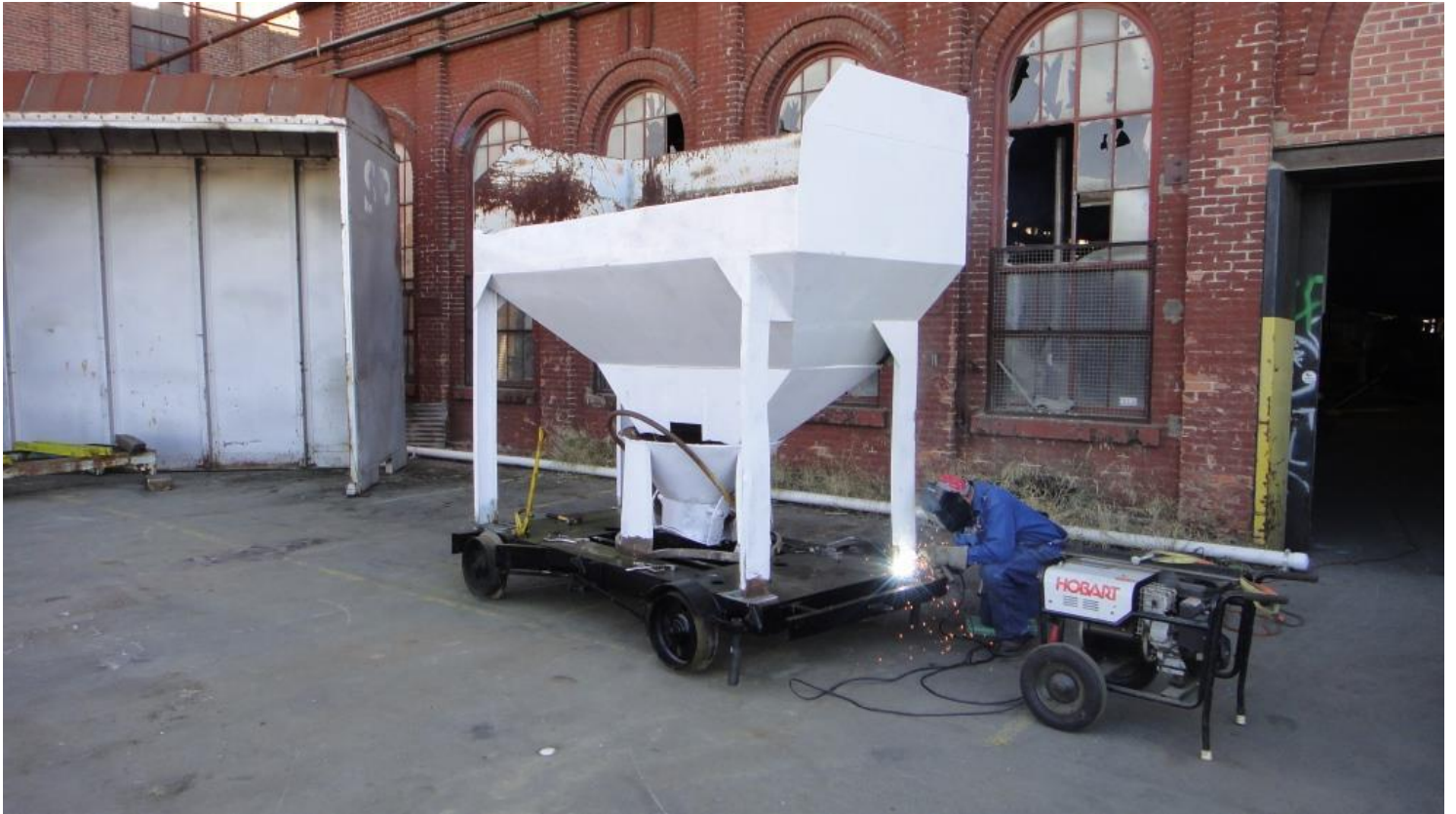
Cliff welds the leg of the new ballast hopper onto its deck
