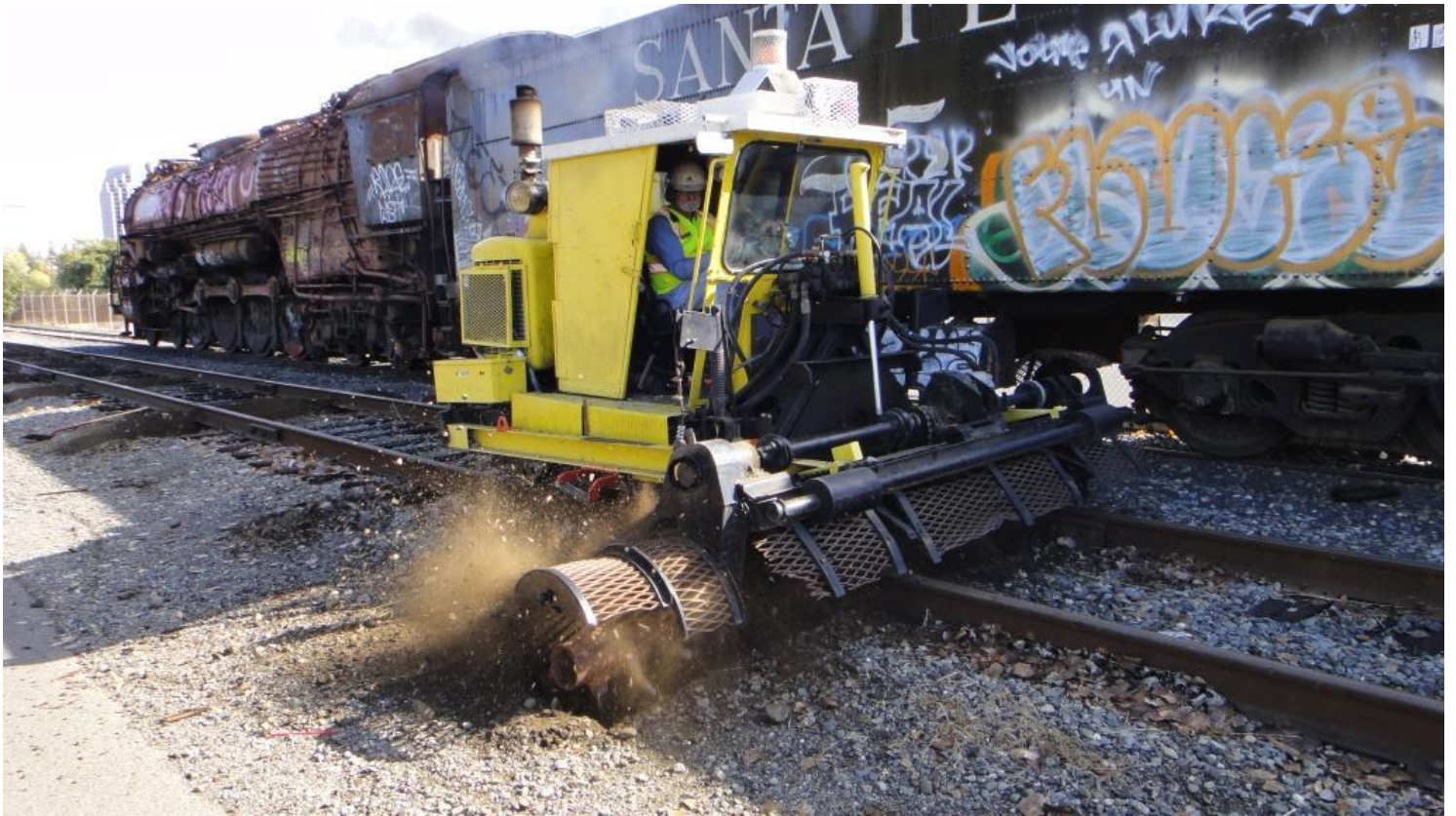
Alan comes through with the scarifer-inserter to dig out the crib of a removed tie
