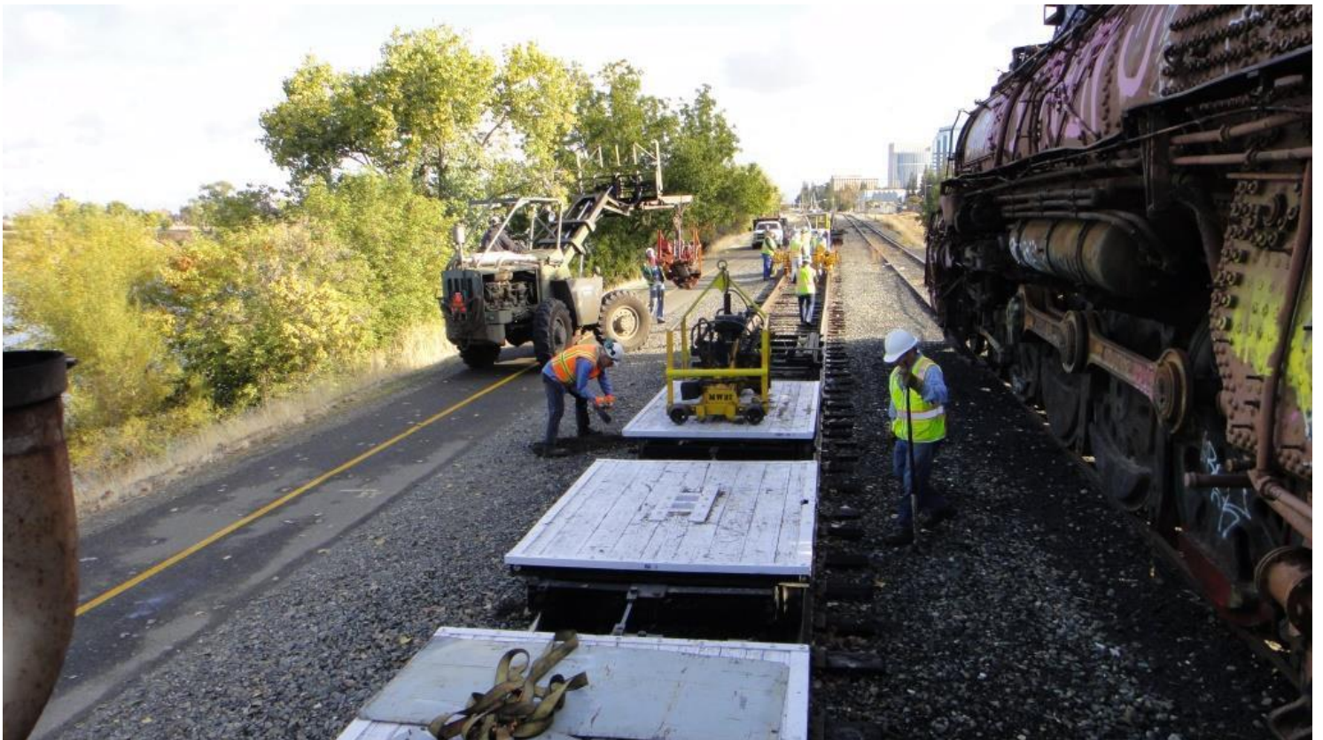
The Team arrives out on the line and begins deploying equipment
