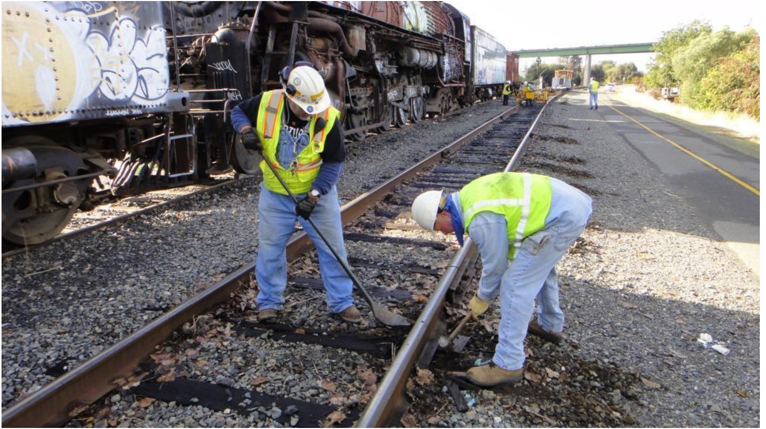
Mike F., and Mike M. remove tie-plates, many of which were cut down into the tie making them difficult to remove
