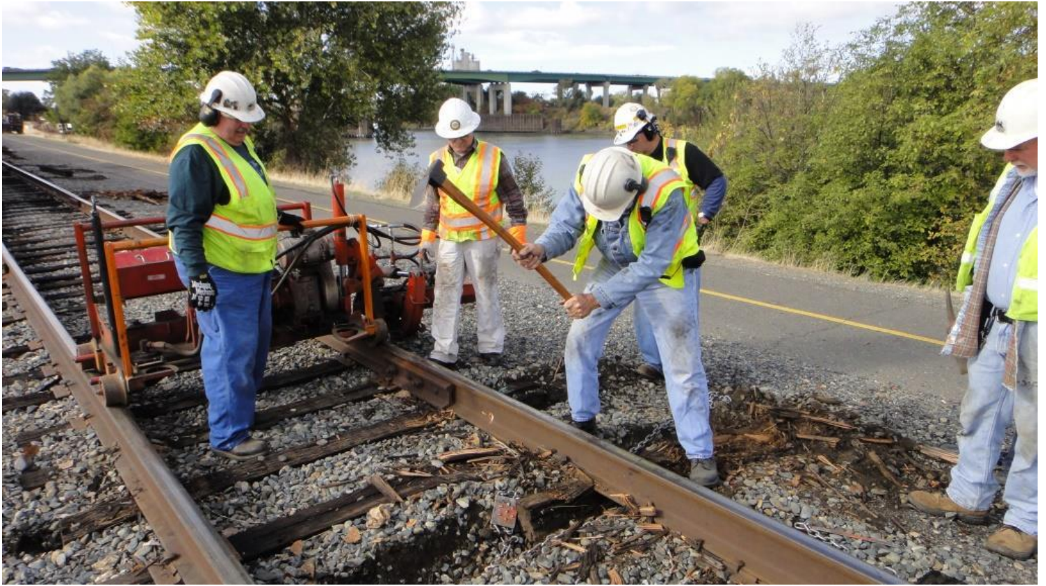
Alan uses an adz to chop away at a plate-cut tie
