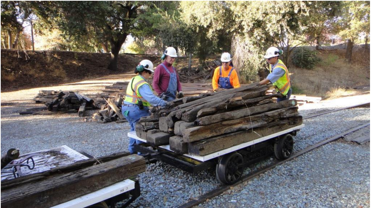
Some whole ties but mostly pieces are added to our dead-tie pile at Setzer by Heather, Steve, Dave, and Matt
