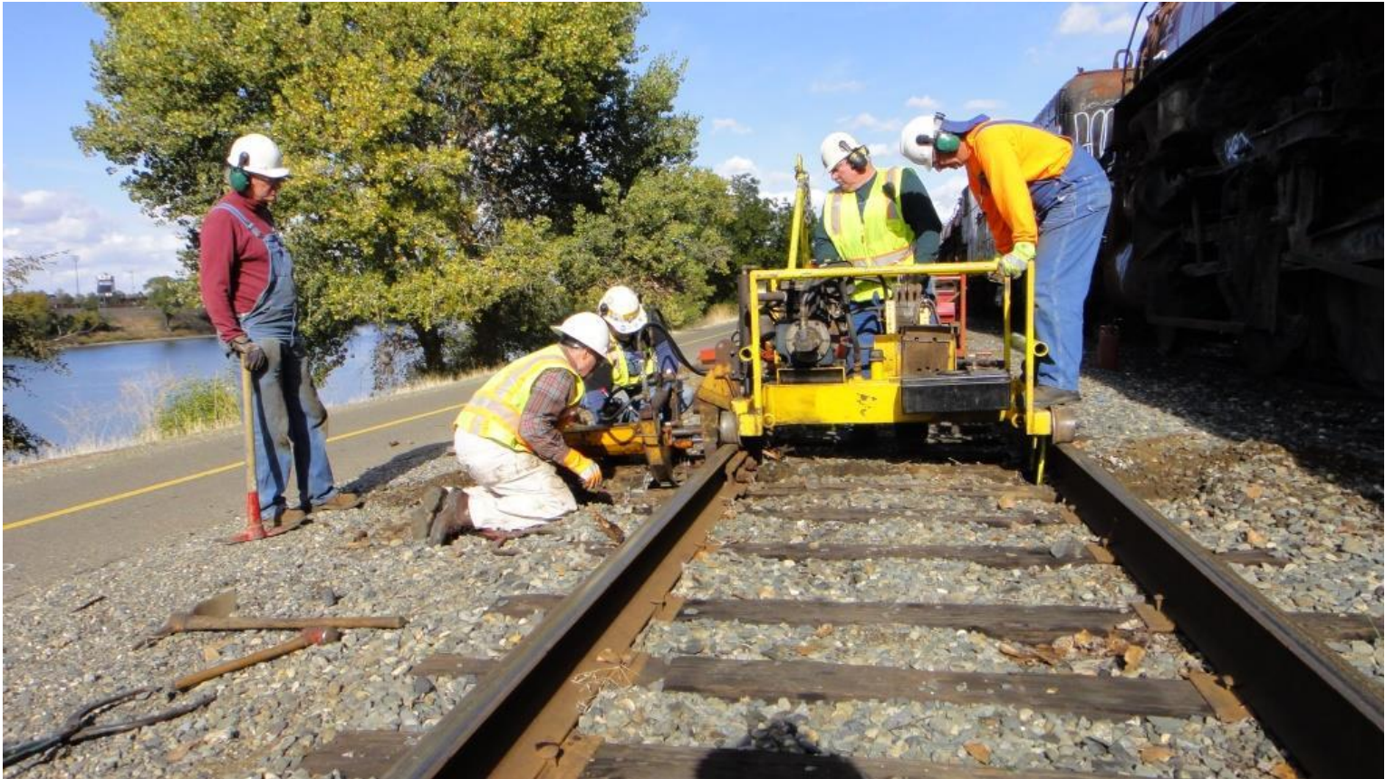
Catastrophe! The hydraulic cylinder that lifts the ram-arm has bent while trying to grab hard-packed tie
